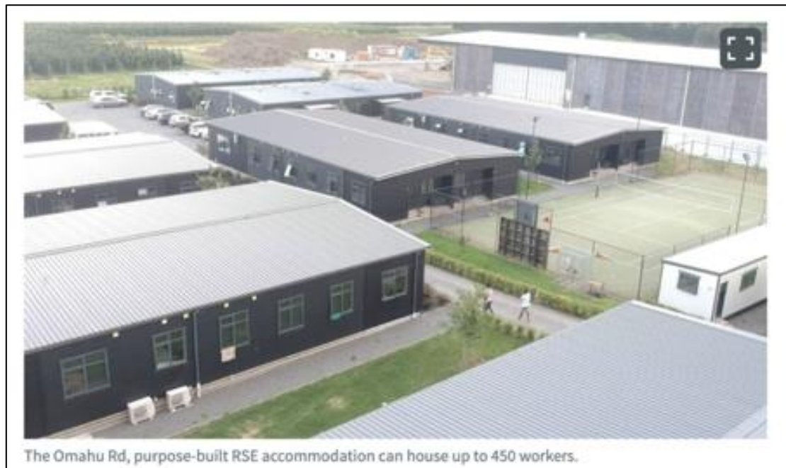
Figure 6.5: Built multi-complex facility in Hastings (Source: Stuff.co.nz Pang 2023)
