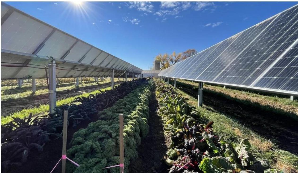
Figure 19. Agrivoltaic solar farm in Colorado (Source: Siegler, 2021).
