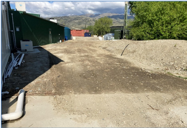
Photo 7: Driveway south of the fruit packing shed, viewed from the north west facing east.
