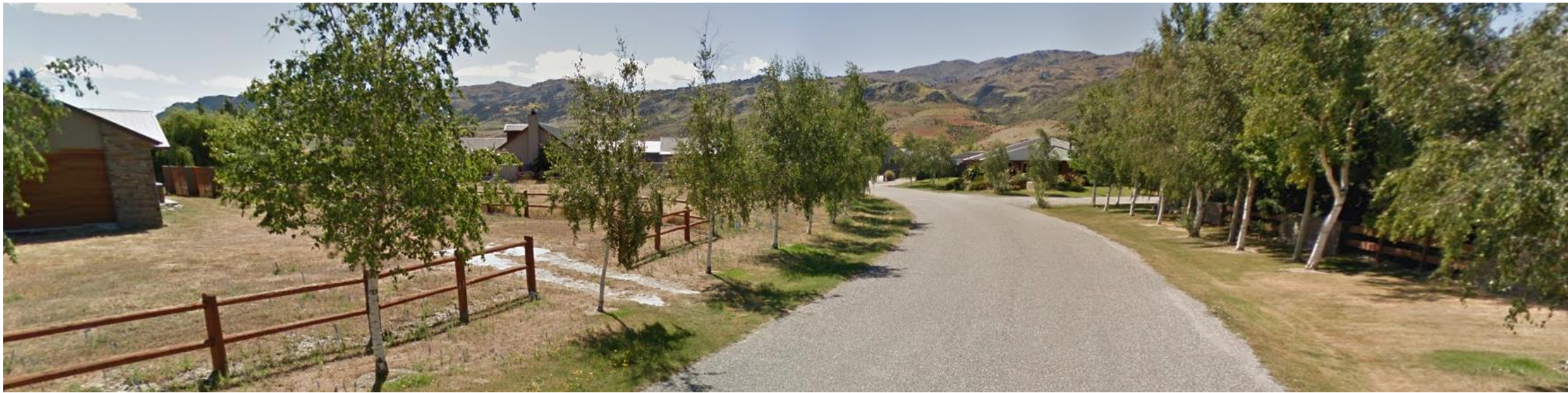
Photograph 8: Typical character of Pisa Moorings streetscape, with street tree plantings, no footpaths, swale drainage, no street lighting and low fencing.
