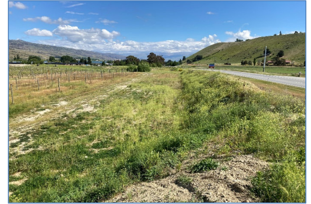
Photo 3: Earth bund west of the vineyard, viewed from the north facing south.
