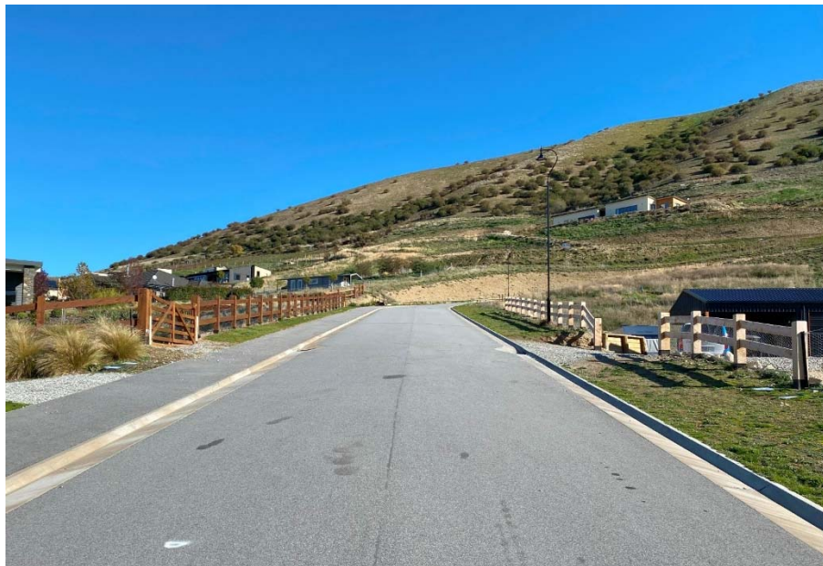
Photograph 3: Turner Terrace Looking West
