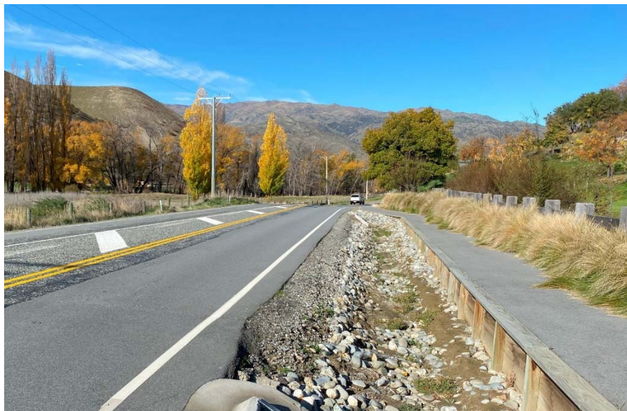
Photograph 6: Footpath on Lowburn Valley Road Just South of Turner Terrace Intersection
