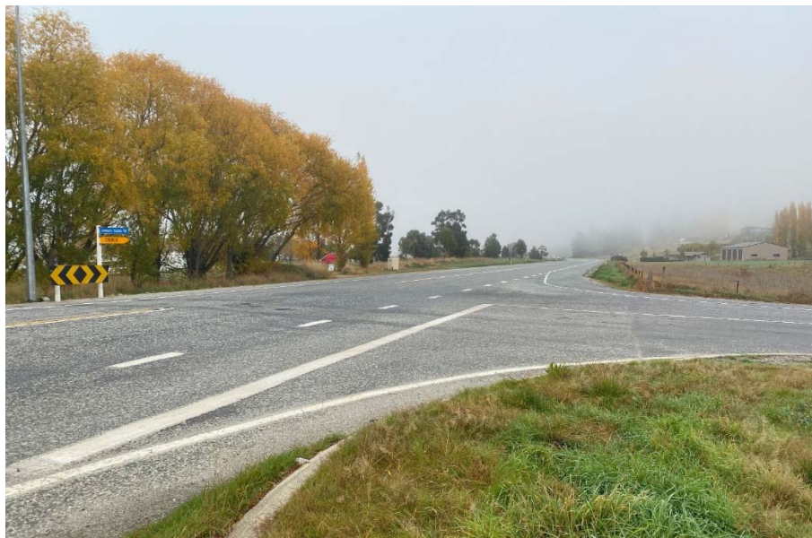
Photograph 5: State Highway 6 / Lowburn Valley Road Intersection
