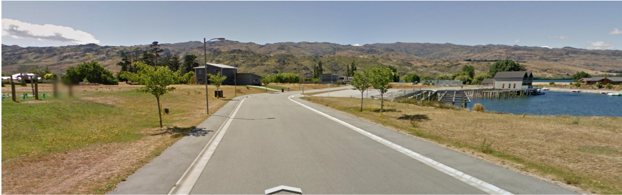
Photograph 11: Typical character of Pisa Moorings streetscape, with limited street tree plantings, footpaths on either side of the street, mountable kerb and channel stormwater management, suburban street lighting and limited fencing.
