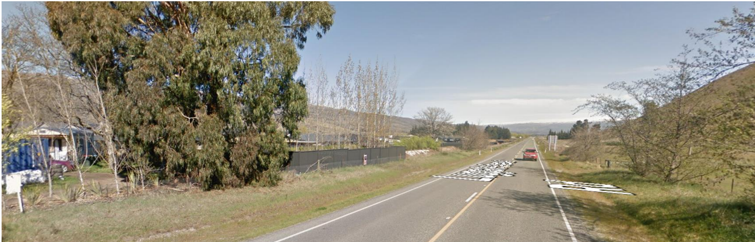
Photograph 7: Typical character of the highway interface with the existing Pisa Moorings development to the south of the site (looking southwards along SH6).
