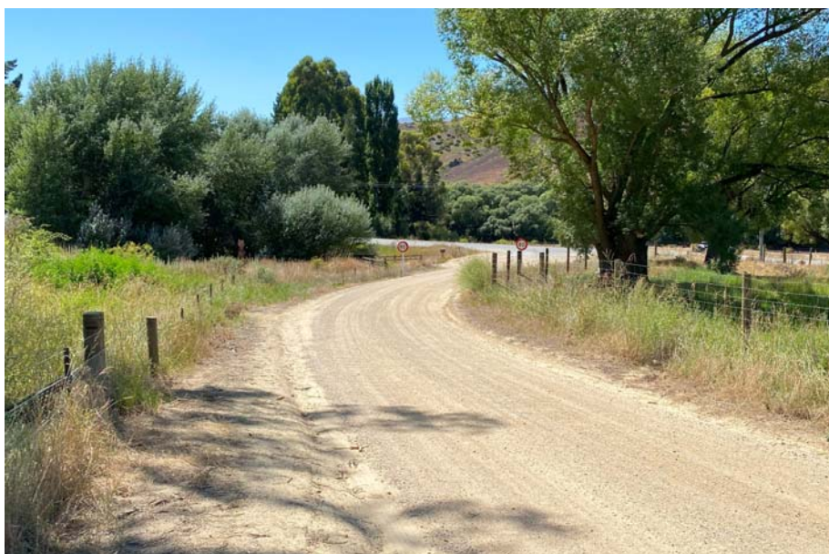
Photograph 1: Schoolhouse Road Looking East (Site on Left)
