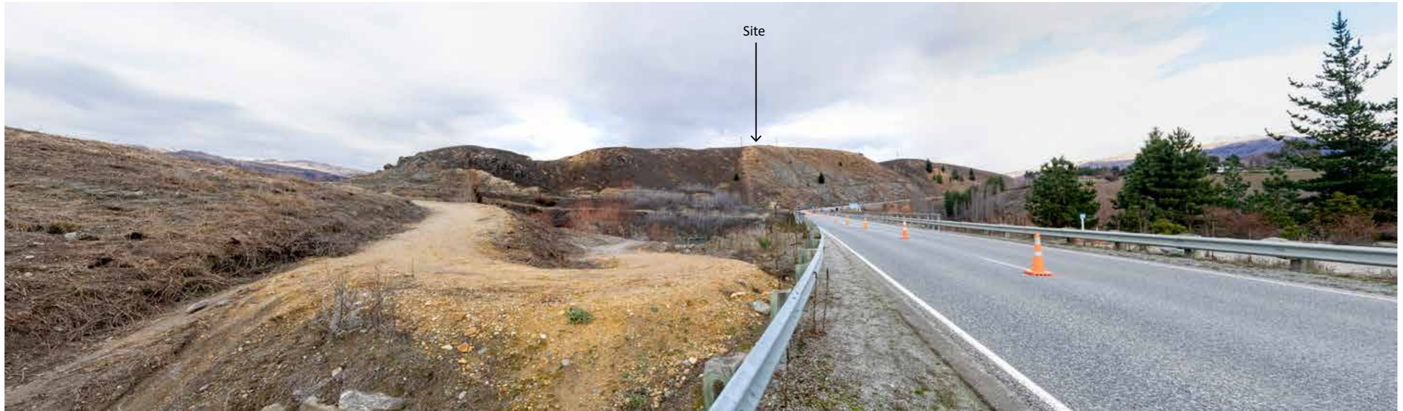
Viewpoint Photograph 1: Kawarau River Bridge Date: 09 July 2020 Time: Between 12:00 and 14:00 Camera: Canon EOS 7D Mark II 30mm Focal Length
