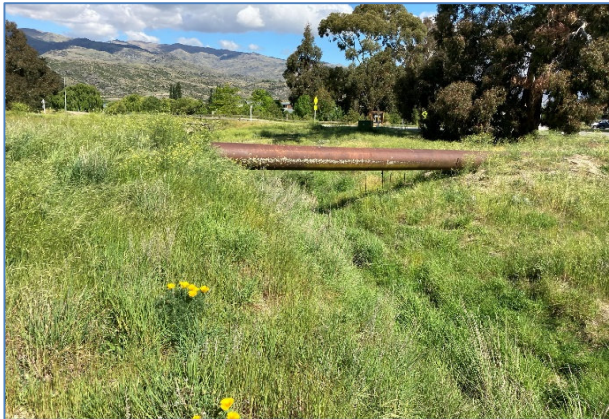
Photo 5: Gully along the southern site boundary, viewed from the north west facing south east.
