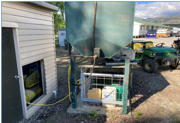
Photo 10: Site surface adjacent to an above ground fuel storage tank.
