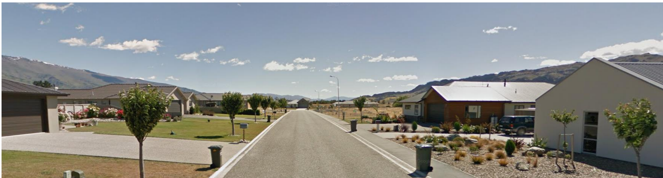
Photograph 10: Typical character of Pisa Moorings streetscape, with some street tree plantings, a footpath on one side of the street, mountable kerb and channel stormwater management, column street lighting and no fencing.
