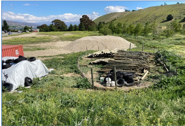
Photo 1: Shipping container, stacked treated timber and soil stockpile in the southern portion of the site.
