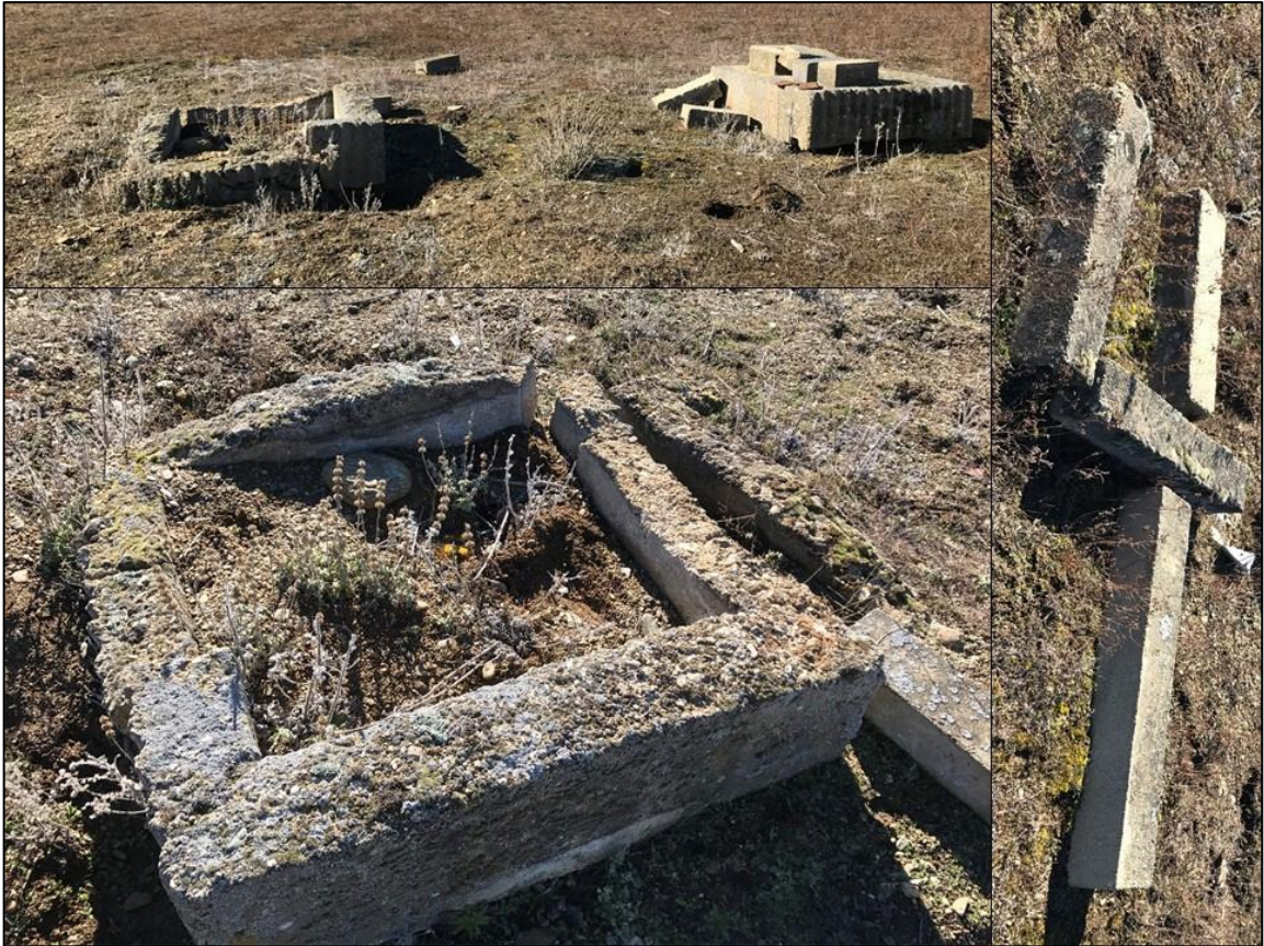
Plate 9: Concrete feature north of miner's residence
