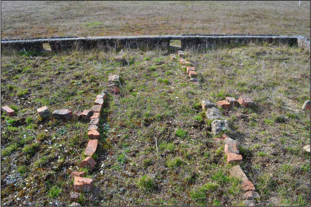
Figure 9. Remains of house sub-floor showing the use of brick to presumably support a suspended timber floor.
