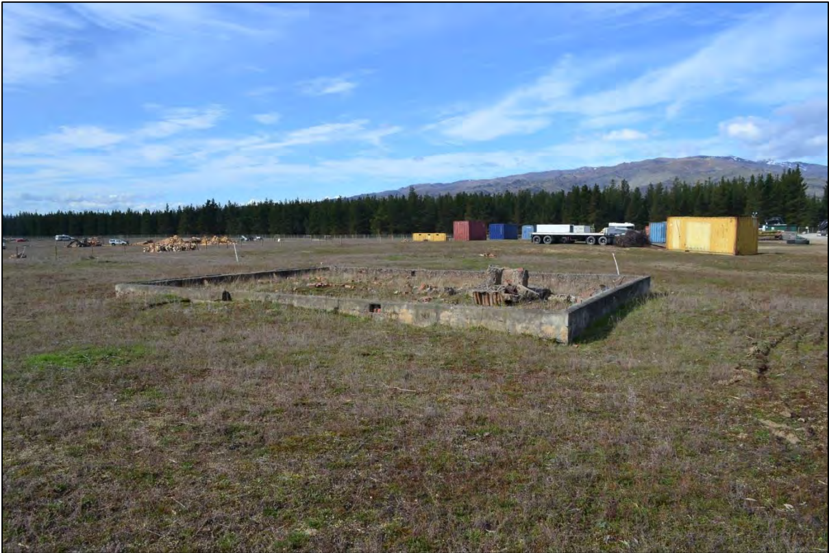
Figure 7. Concrete house foundation located near the southern boundary (see Figure 5).
