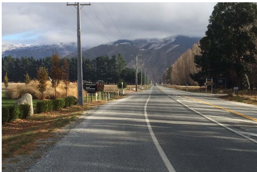
Photograph 8: Wide Shoulder on Southern Side of Highway (Looking West towards Sandflat Road)
