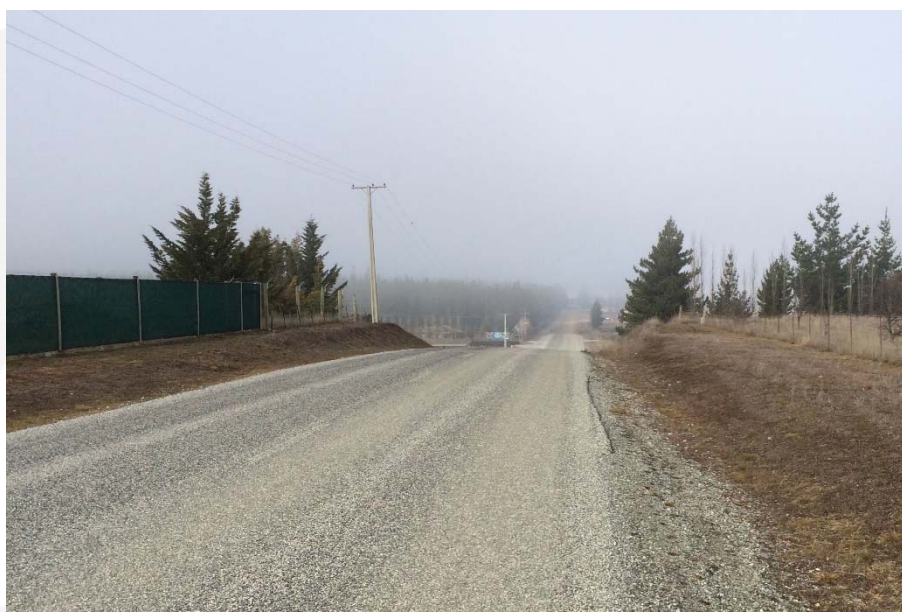
Photograph 2: Sandflat Road South of Highlands Motorsports Park, Looking South
