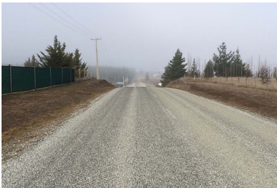
Photograph 3: Crest Curve in Sandflat Road 360m South of State Highway 6, Looking South
