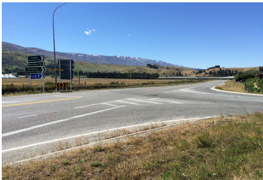
Photograph 10: State Highway 6 / McNulty Road Intersection, Looking North
