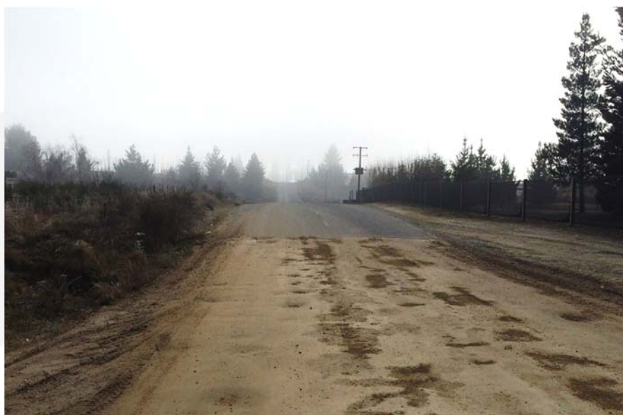
Photograph 4: End of Seal in Sandflat Road, Looking North
