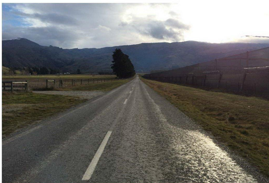
Photograph 1: Ripponvale Road Looking West, Towards Site
