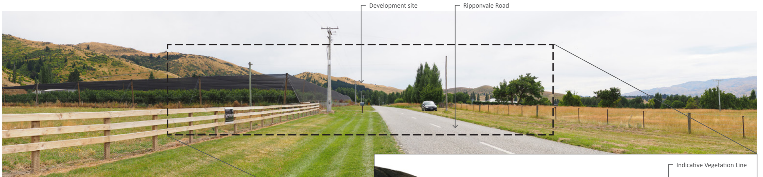
View 01: View from the north-south limb of Ripponvale Road Distance: 400m Date: 29-01-2019 Time: between 12-2pm
