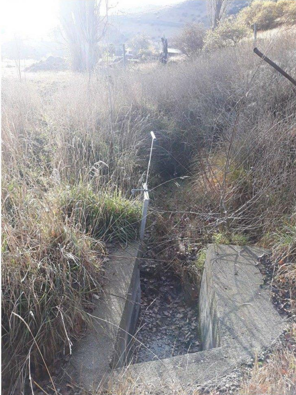
to NZCC supply channel
