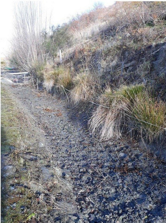
Stock grazing race side vegetation and defecating in the basin of the B race
