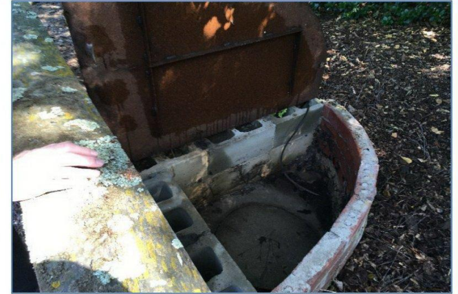
Photo 21: Underground water storage tank, south of the dwelling on the southern property.
