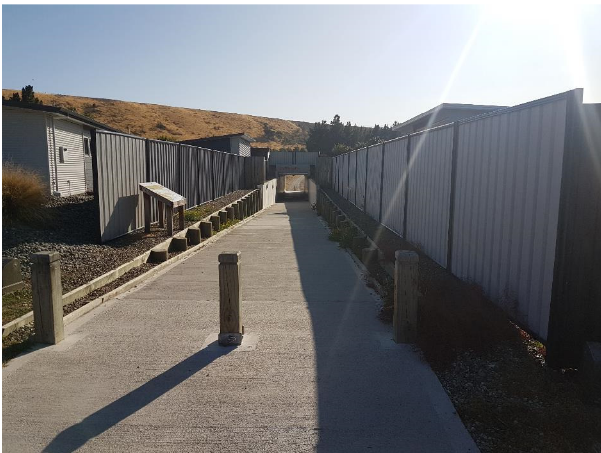
Figure 2 Albert Drive Active Mode Underpass
