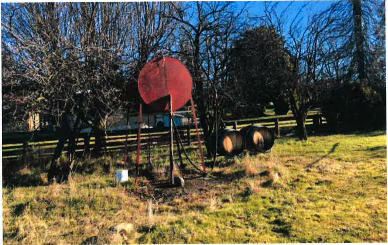
Above ground fuel storage tank.
