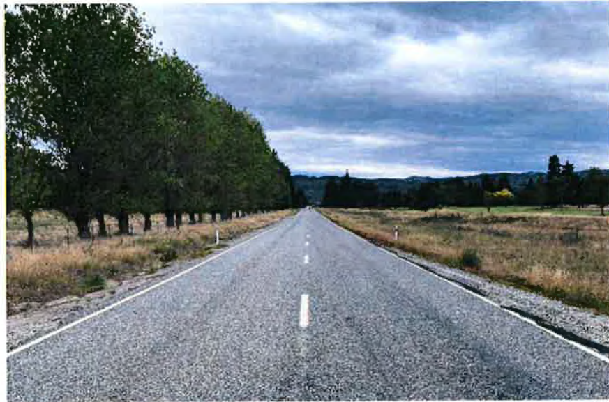
Photograph 1: Dunstan Road Looking South (Site on Left)
