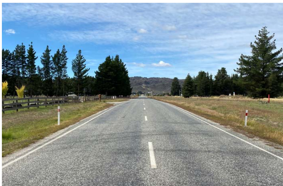
Photograph 1: Dunstan Road Looking South
