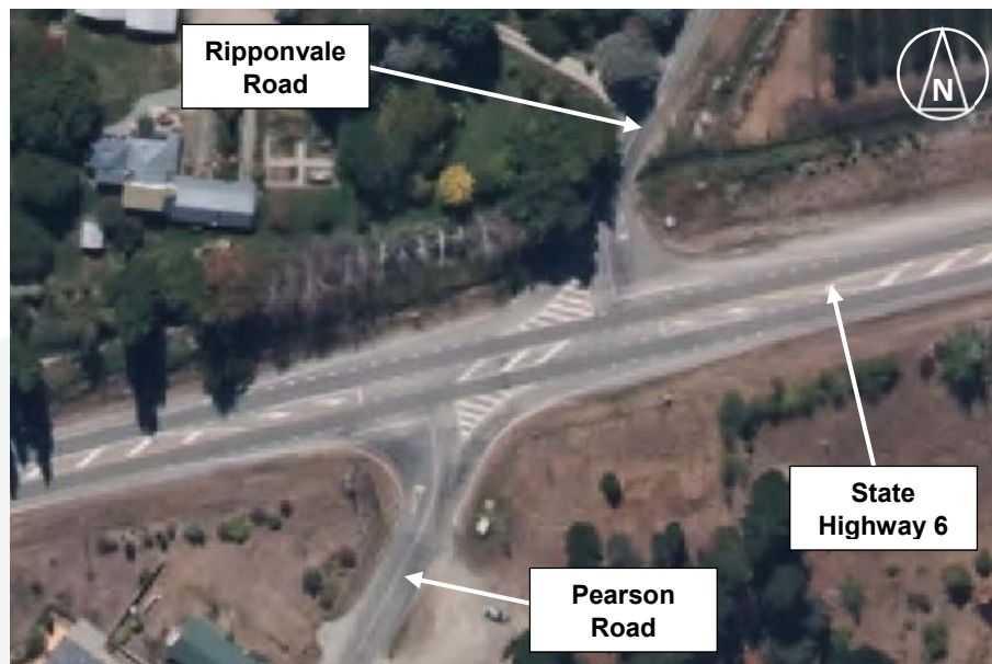
Figure 1: Aerial Photograph of State Highway 6 / Ripponvale Road Intersection
