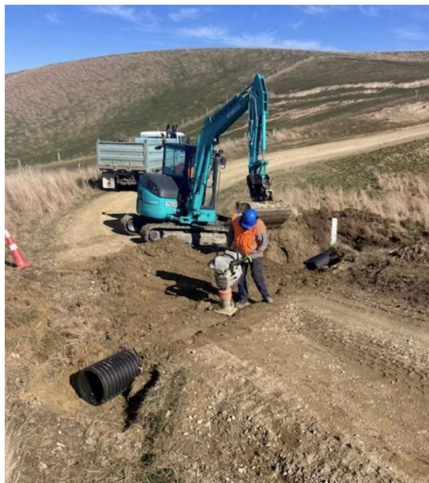
Culvert replacement Three Brothers Road
