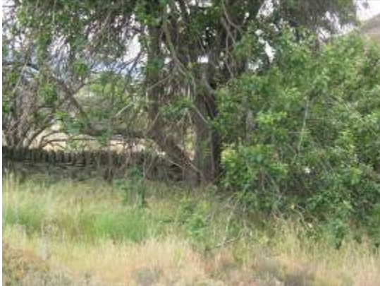
Photo V1 Damage to walls
