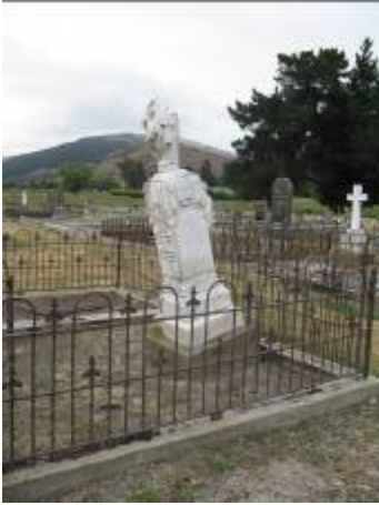
Photo T1 – Ornate headstone on lean owing to ground slumping
