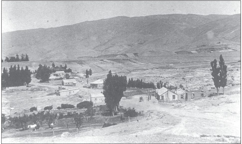
Figure 14. Bannockburn c. 1899, looking southwest from Slaughteryard Hill. Bannockburn Hotel on the right. Note extensive sluicings behind. Mrs E. Olds, Cromwell, P. Crump Collection.
