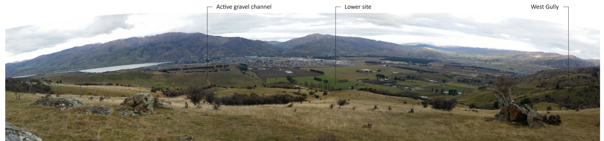
View 09 - View from Northwest hillside toward lower site and neighbouring properties to the Southeast.
