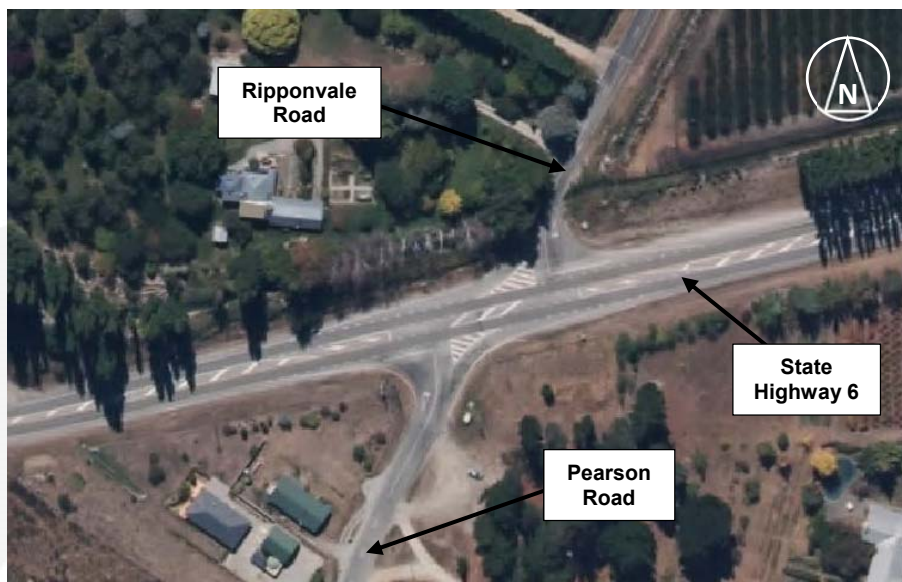
Photograph 5: Aerial View of the State Highway 6 / Ripponvale Road / Pearson Road Intersection
