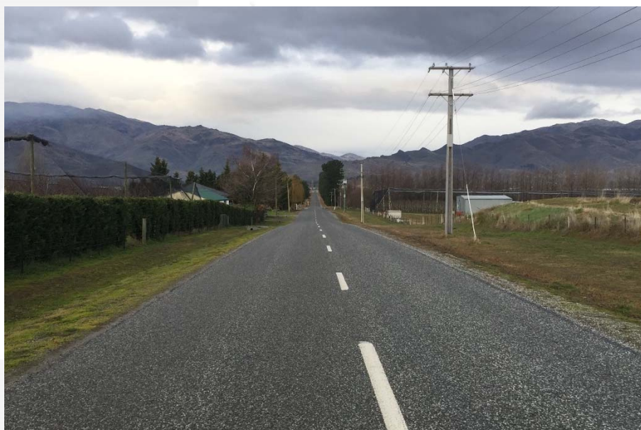
Photograph 1: Ord Road Looking East
