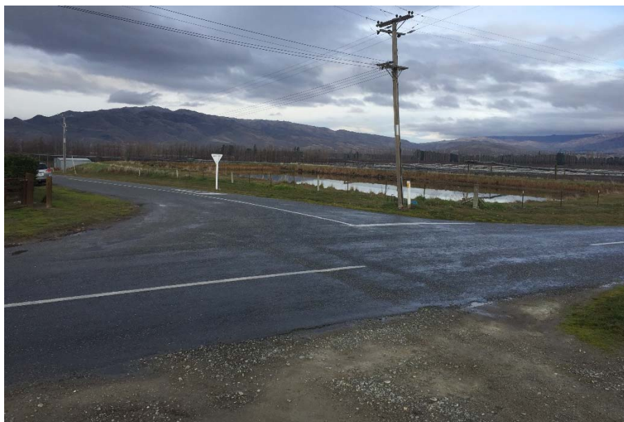
Photograph 4: Ripponvale Road / Ord Road Intersection Looking South
