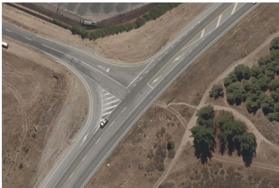
Photograph 2: Aerial Photograph of State Highway 6 / Ripponvale Road Intersection
