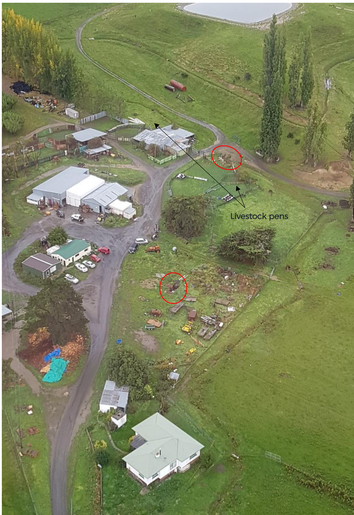
Central area of site showing packing sheds, disposal pits (circled) and deposited materials
