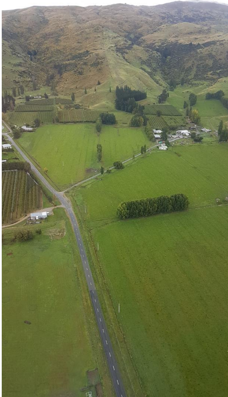
Western part of site with Ripponvale Rd in foreground
