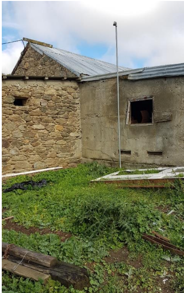
Location of buried fuel storage tank
