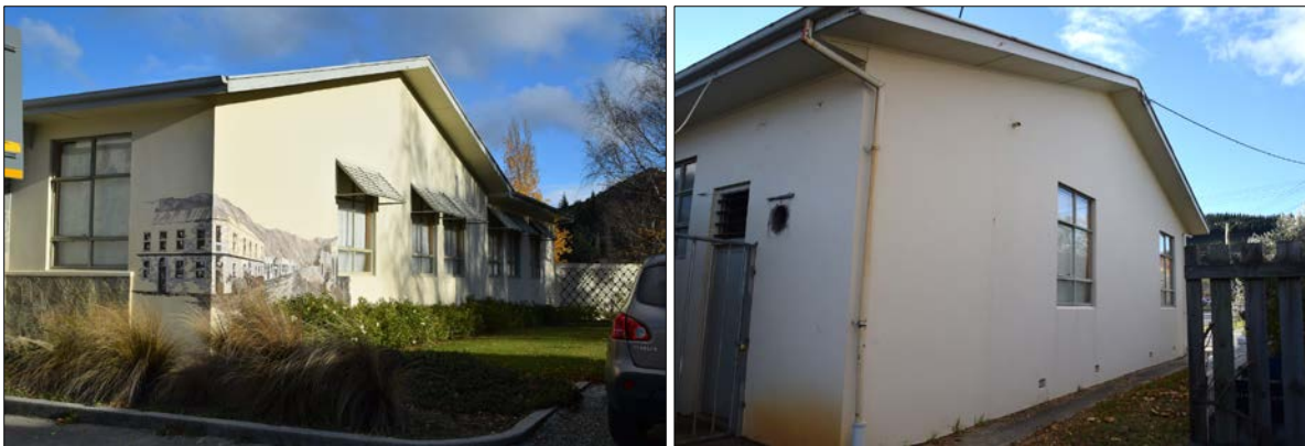
Figure 5: The north-west elevation of the museum with the Clyde mural c. 2007 (left); the south-east elevation (right).
