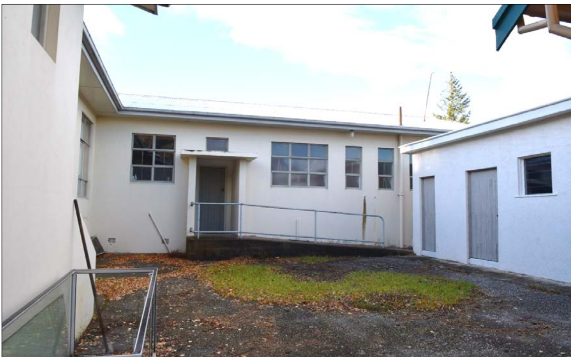
Figure 7: The rear, south-west elevation with the Ablution Block to the right of view (c.1965) and the return west wing to the left.
