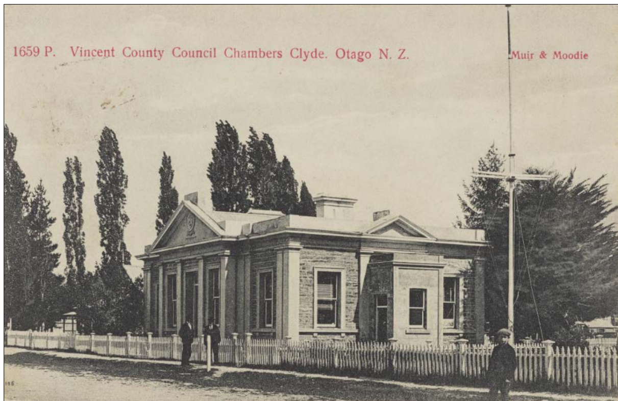
Figure 22: A view of the County Chambers taken c.1905 by Muir & Moodie showing the handsome stone building with its classical architectural detailing. Image: Museum of New Zealand/Te Papa Tongarewa, MA_1407409
