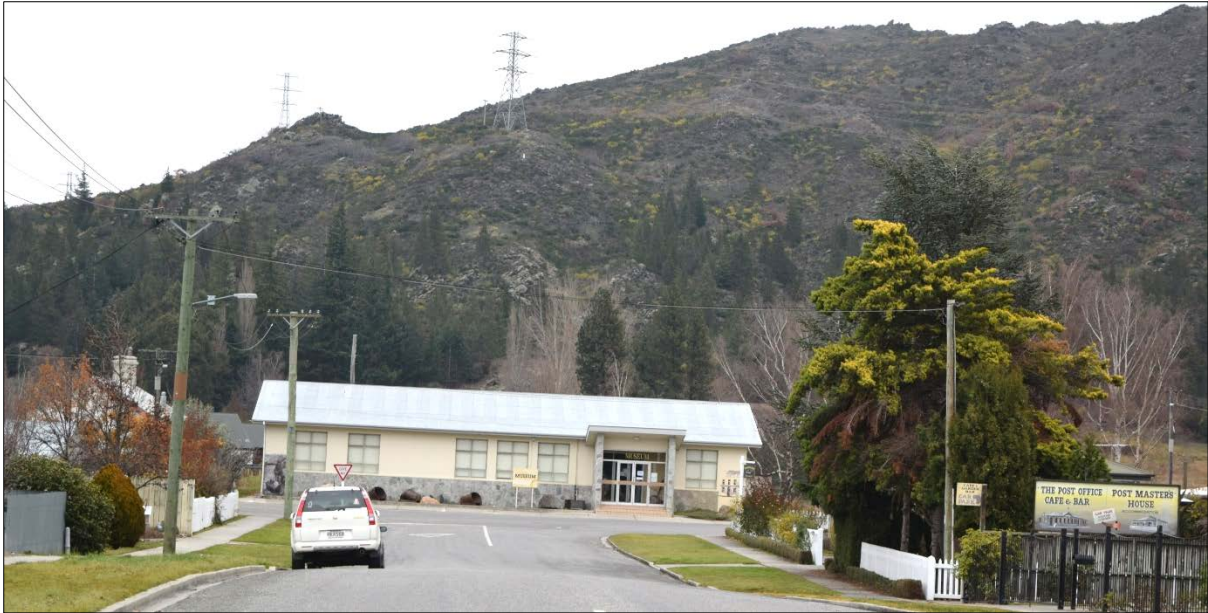
Figure 15: The setting of the Blyth Street Museum site (winter view).
