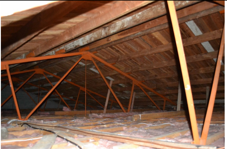
View of roof void from the access hatch
