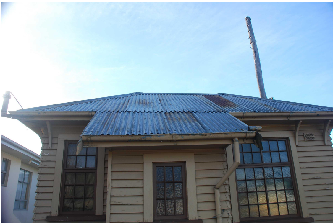
Figure 26 The rear roof slope clad with galvanised steel sheets.
