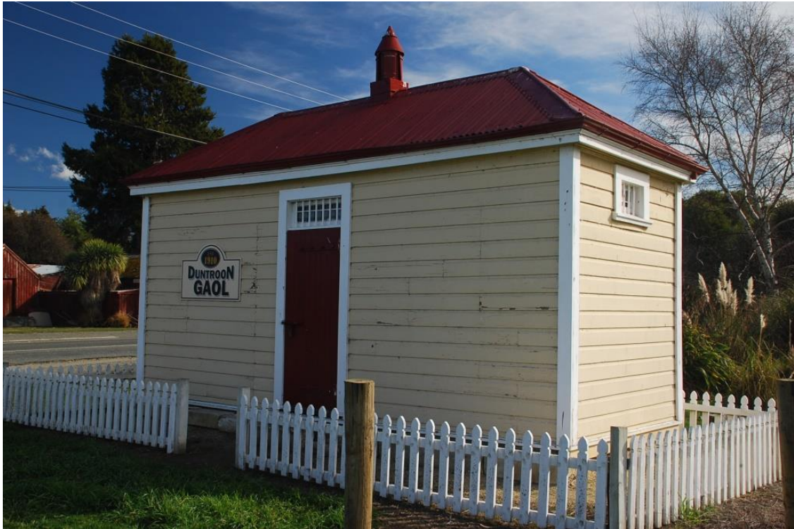
Figure 12 The lock-up or gaol at Duntroun c. 1910. Note the high level barred windows and roof vent. Jackie Gillies + Associates 2009.
