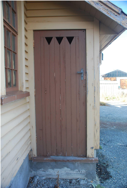
Figure 22 The vented door to the WC.
