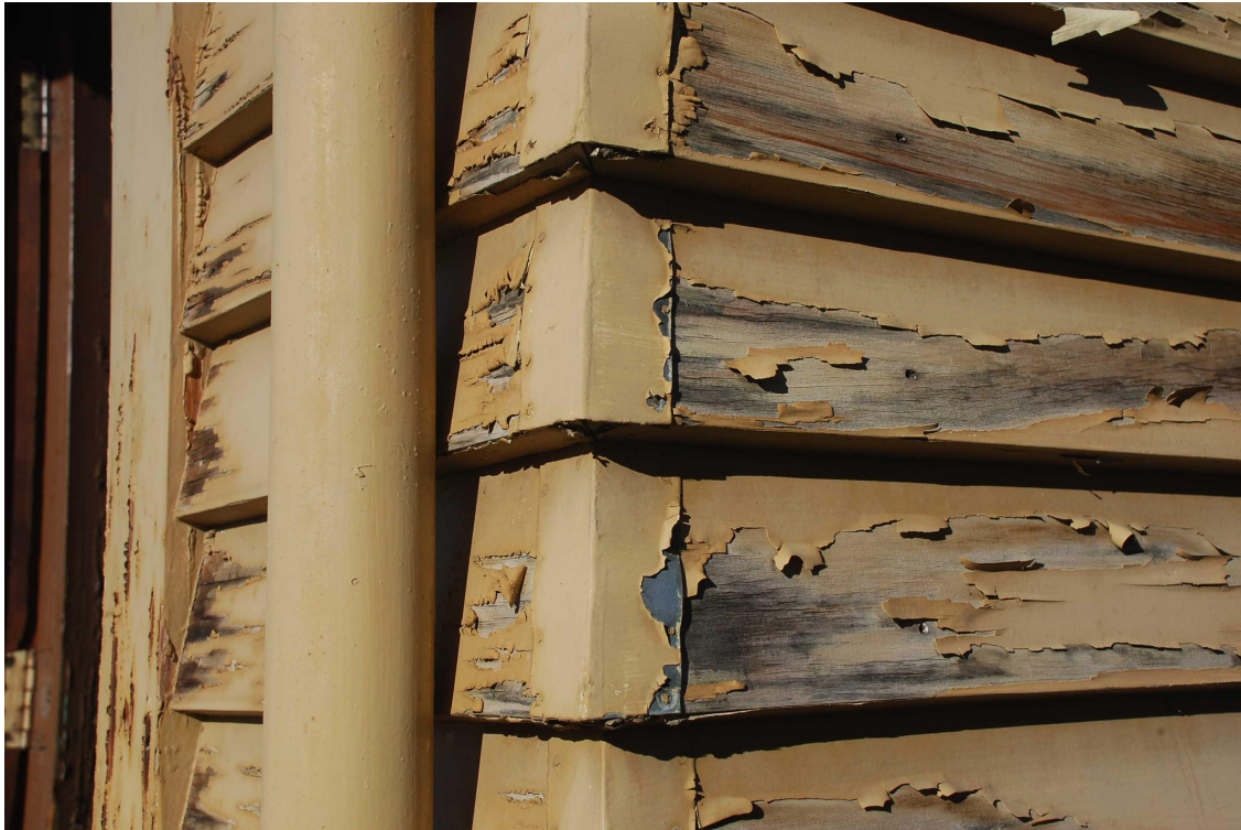
Figure 25 Galvanised steel strips to the mitred corners of the weatherboards.
