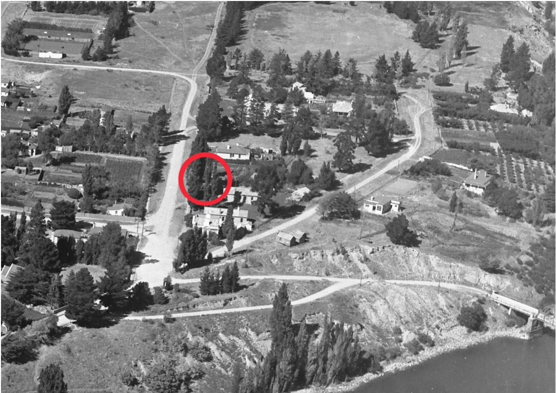
Figure 4 This photograph (ref: 03 CEO1-38 - 0014 VC Browne & Son – Clyde) was taken at the same time as the one in Fig. 3 above and the Lock-up (approximate location circled) is concealed in the trees fronting Blyth Street. The photograph does however show the Sergeant's House much more clearly (at roughly 4 O'clock on the red circle).
