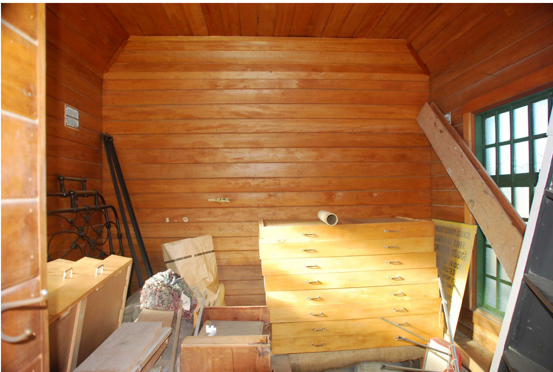
Figure 28 The interior of the cell from the cell doorway.
