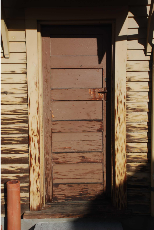
Figure 21 The entrance door leading to the lobby.
