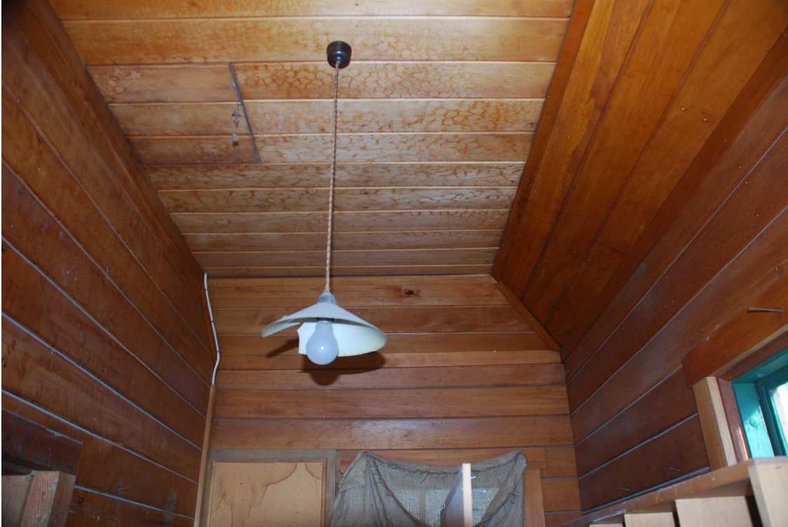
Figure 29 Tongue & groove ceiling and wall linings in the lobby.
