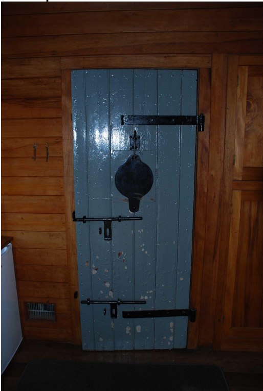
Figure 15 The timber and steel cell door at St. Bathans' lock-up – by kind permission of Angela Middleton and Ian Smith. Jackie Gillies + Associates 2014.
