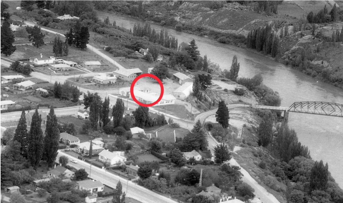
Figure 6 This aerial was taken in 1965 (ref: 04 9525 - 9552 VC Browne & Son - Clyde). The trees lining Blyth Street have gone and Pyke Street has been built. The Sergeant's House remains (at about 10 O'clock just outside the red circle) and, by this year, the Police Lock-up has been relocated to the Courthouse site. It appears to be visible in the centre of the circle at the rear of the Courthouse. With close scrutiny of the photograph the hip of the roof can be seen and the large window on the side of the lobby.
