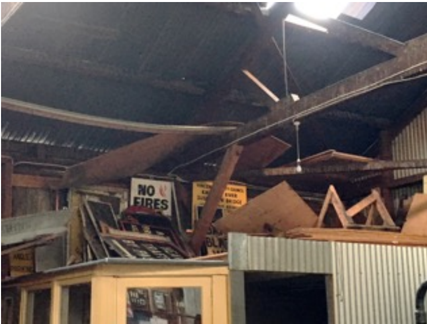
Image: Storage area above the smoko room, as surveyed.
