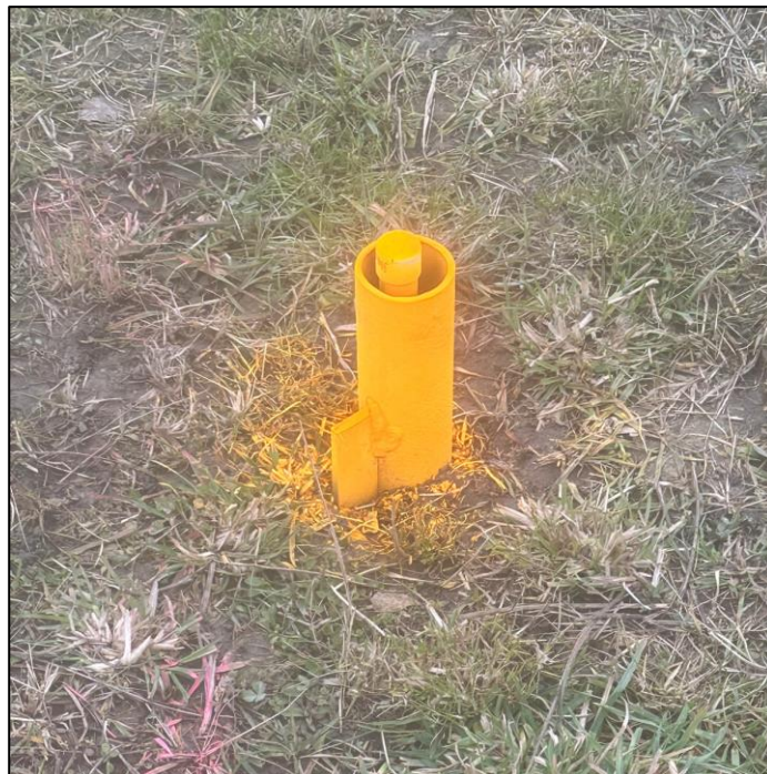
Figure 13 Photo of piezometer (source; HML).
