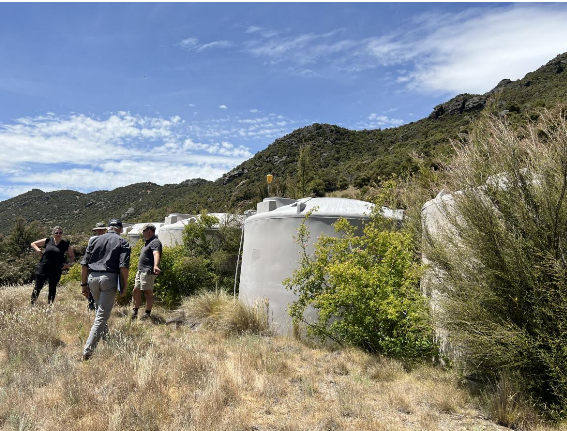
Figure 10: Existing header tanks supplied by Chinamans Terrace Scheme (4 x 25,000L) (14/12/23)
