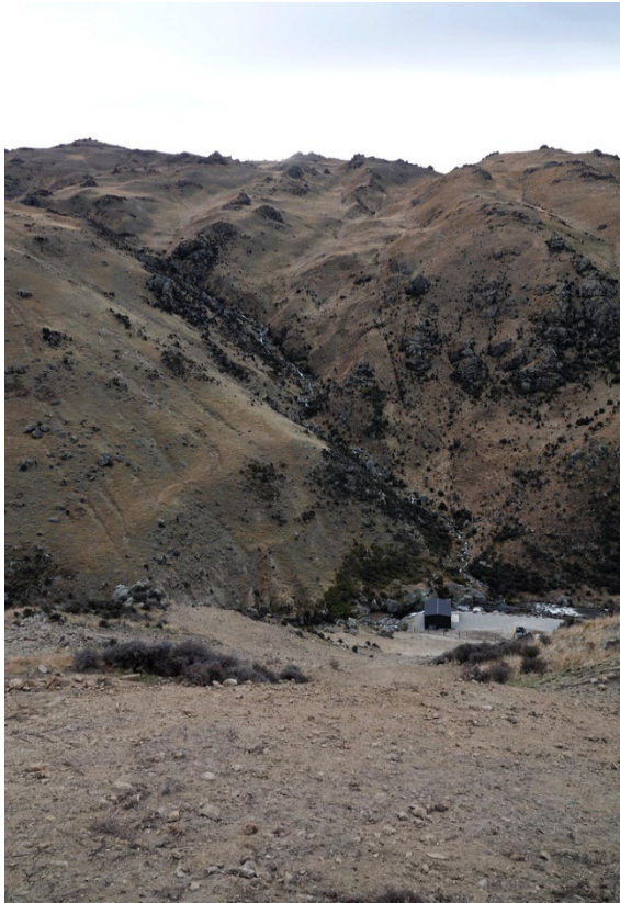
Steep Slope above powerhouse – 2019
