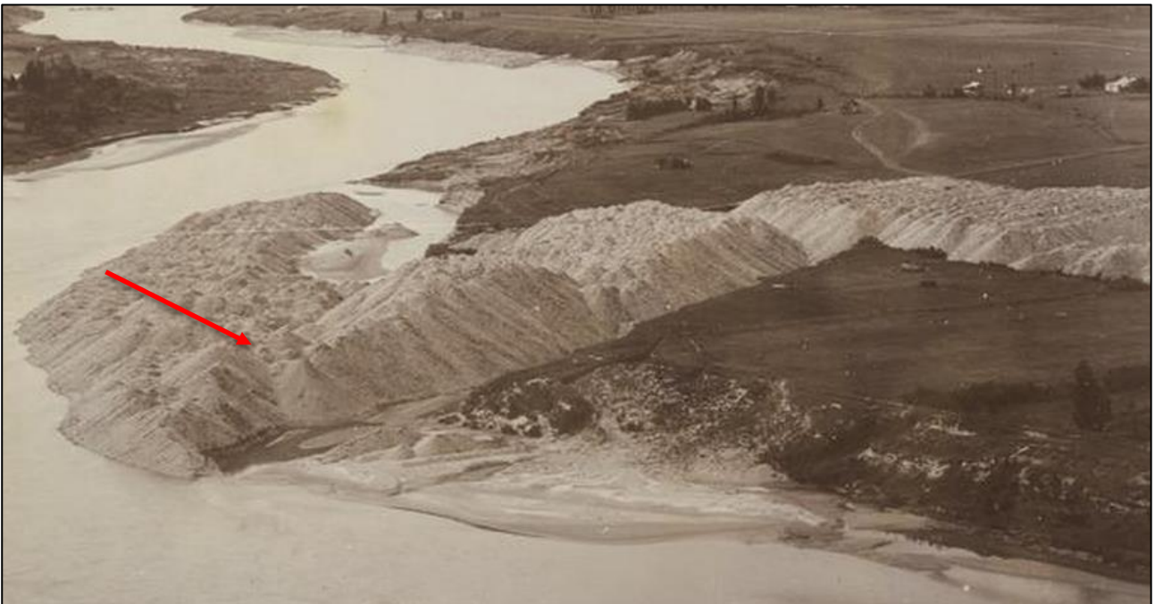
Figure 5-76. Photograph showing the dredging through the project area by 1903, through the location of Henry Raynor's building (the approximate location shown by the red arrow (Unknown, 1903a).
