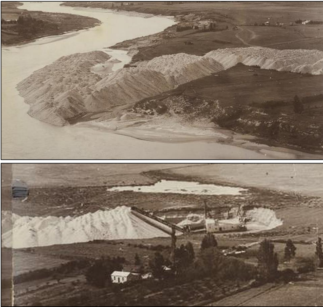
Figure 5-48. Part 1 (top) and 2 (bottom) of the panorama showing the dredging through the project area, in particular Sections 93-95 around 1903. Note the Golden Bed Dredge at the head of the worked area (Unknown, 1903a, 1903b).
