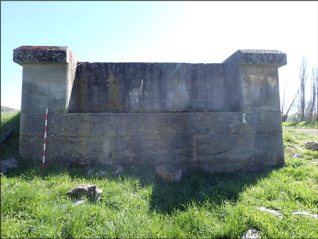
Figure 5-107. Concrete support for railway bridge (POI 12; facing north)
