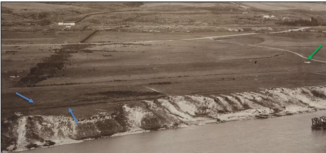
Figure 5-57. Part 3 of a panorama showing the project area from around 1903 showing the Bennet and Company dam (green arrow) as well as both Bennet and Company, and Kitto's water races (blue arrows) (Unknown, 1903c)
