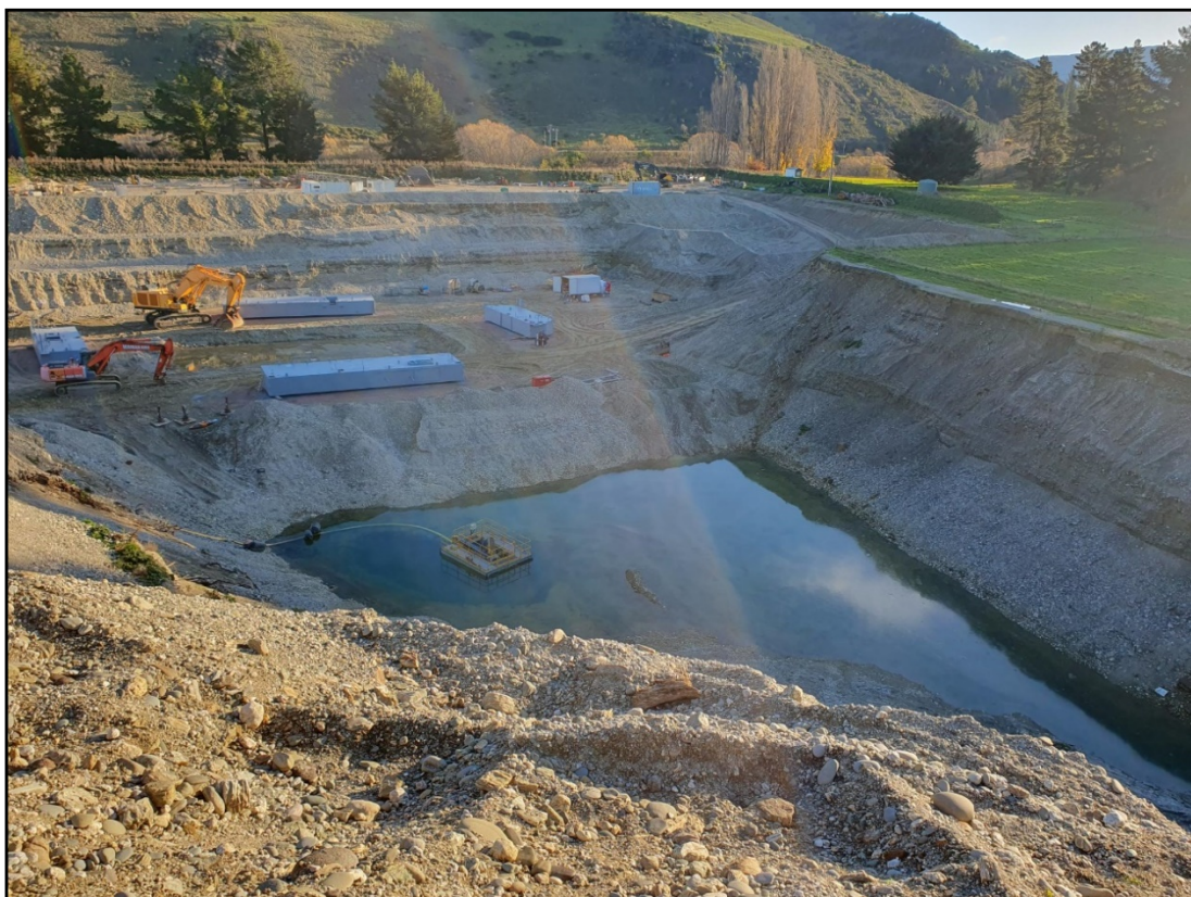
Figure 5: Works already undertaken on the site. Source: Council compliance site visit photos taken on 15 May 2023.
