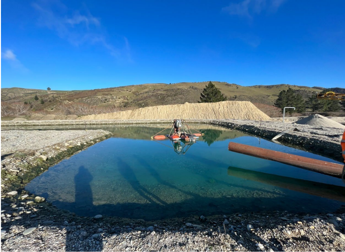
Figure 7: Sediment pond. [Source: Site visit].
