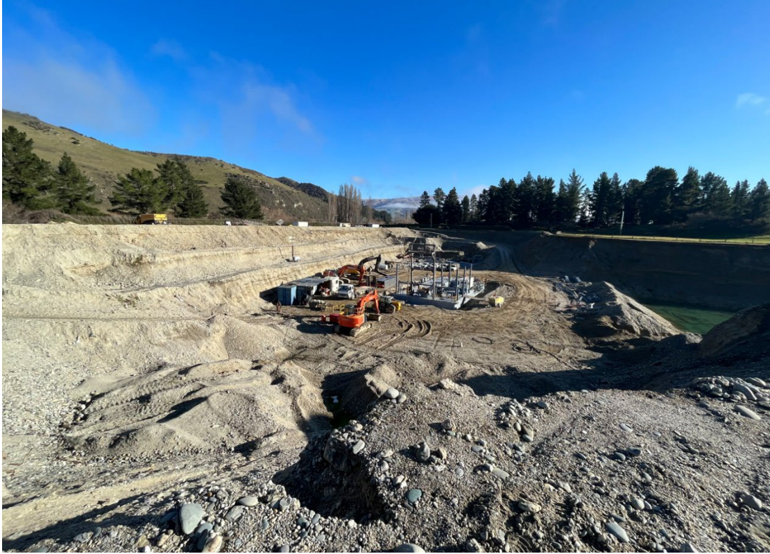
Figure 6: Mine pit, with pond pictured on the right. [Source: Site visit].
