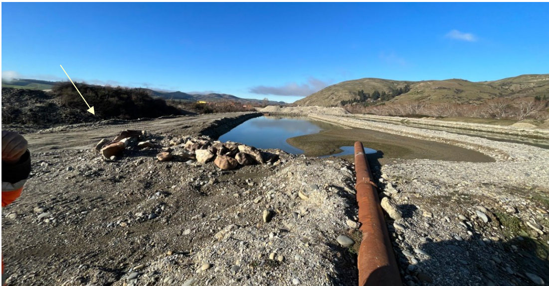
Figure 8: Sediment pond. Discharge area is located to the left (indicated by arrow), away from the Clutha River [Source: Site visit].
