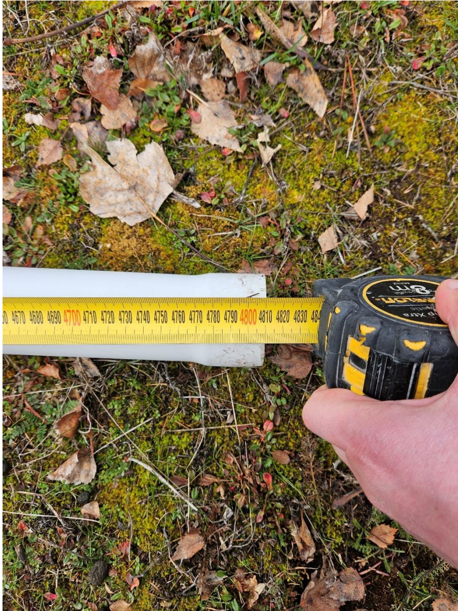
Figure Three: Measurement of smaller poles that were visible standing on the site.
