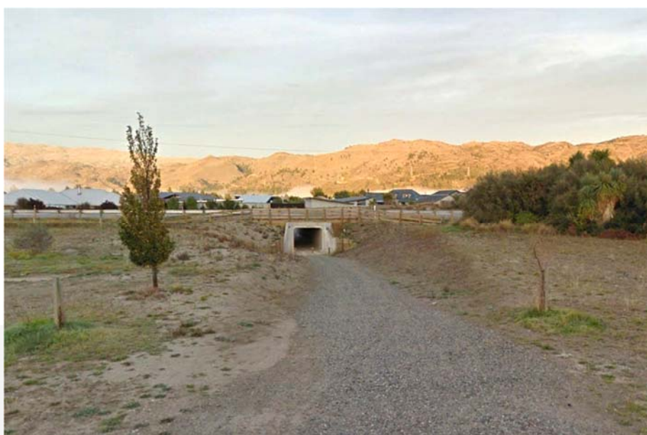
Photograph 7: Underpass below State Highway 8
