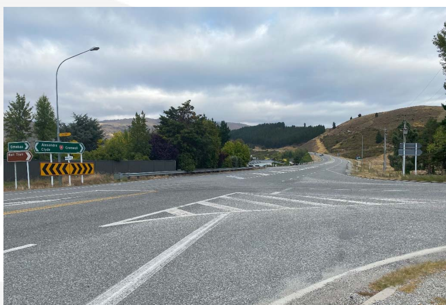
Photograph 6: State Highway 8 / Springvale Road Intersection Looking North
