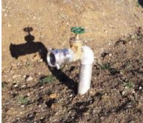
Figure 2: Upstand 100mm Female Suction Coupling
