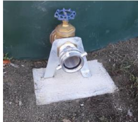
Figure 3: 100mm Female Suction Coupling
